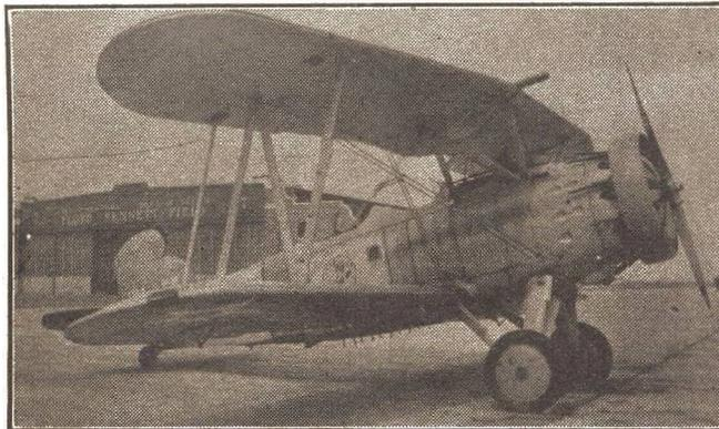
PRESENTING Curtiss' new Helldiver F8C-4 now being used for dive bombing by several Navy squadrons. This "shot" is interesting, since it shows the upper-wing gun and the special bomb racks fitted beneath the wing.
