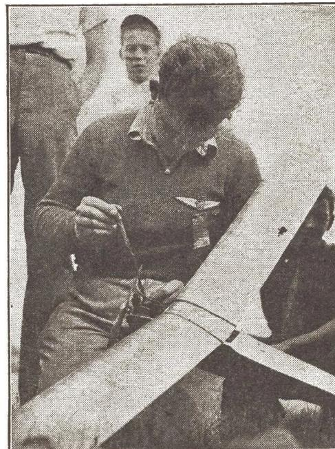
Eye-droppers are standard equipment with all gas jobbers. Above we see Ira Hassad, of California, feeding his tiny 1/2-inch bore engine with one. Ira designed and built this unusually small plant. The model in which it is mounted carries 300 square inches of wing surface.
